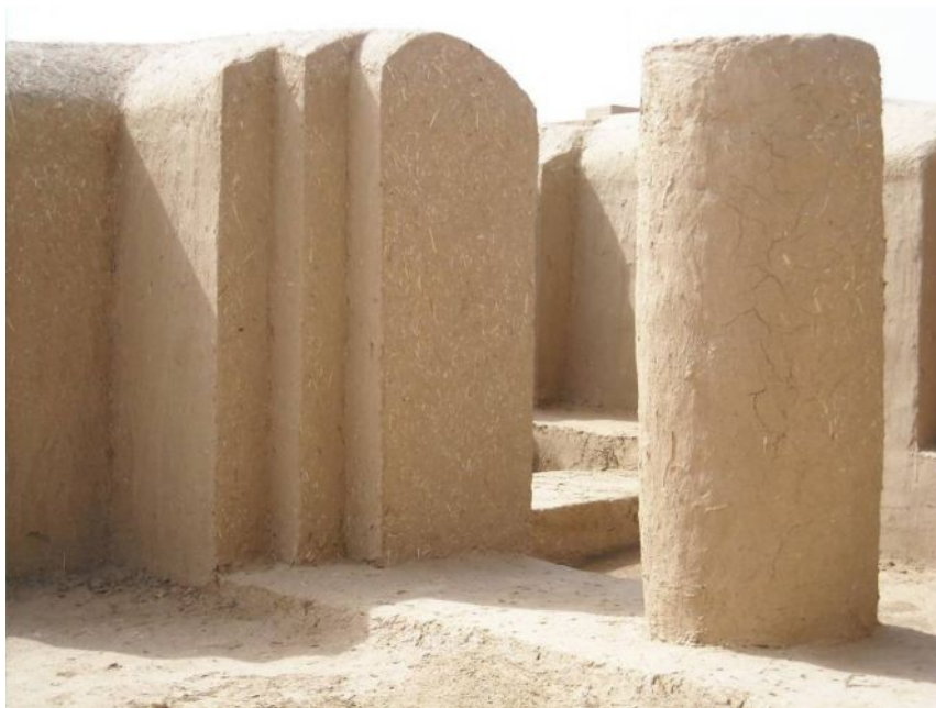
26. Palace. Conservation of the walls. Imitation of wood columns.
